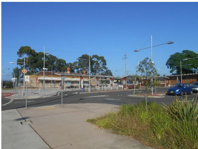
Existing Windsor Railway Station and Bus Interchange
